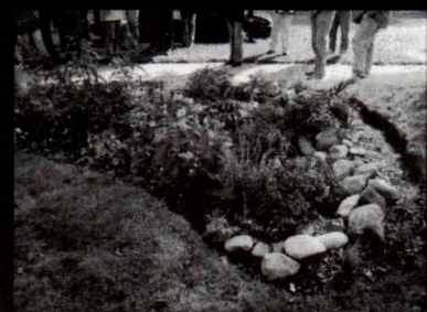
Rain gardens and bioswales are effective ways to manage and clean storm water on-site.
