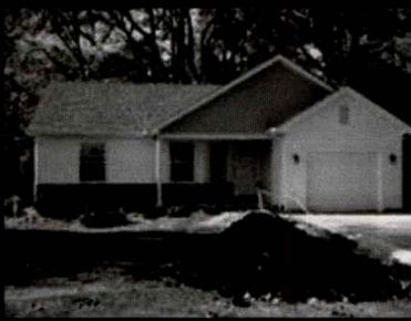
This is an example of a Habitat for Humanity, Porter County, home nearing finished construction.
