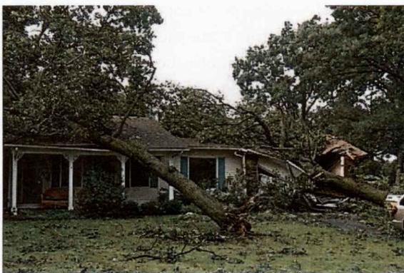
Figure 3-19 Home Damaged During Windstorm
