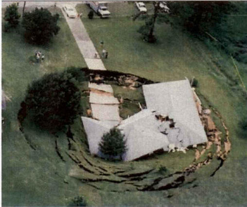
Figure 3-20 Home Swallowed by Land Subsidence
