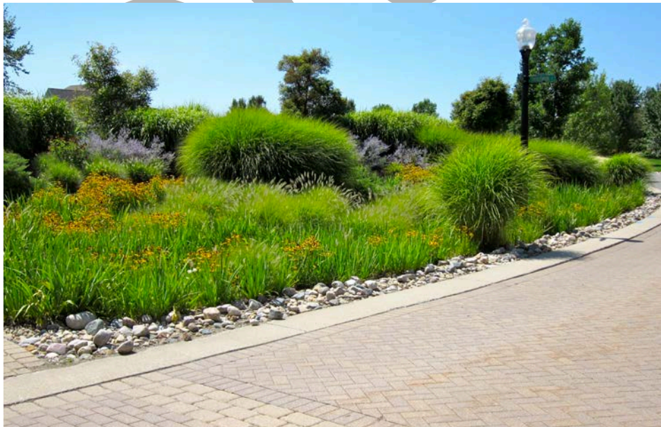
Figure X-8: Infiltration Trench along Curbless Street
