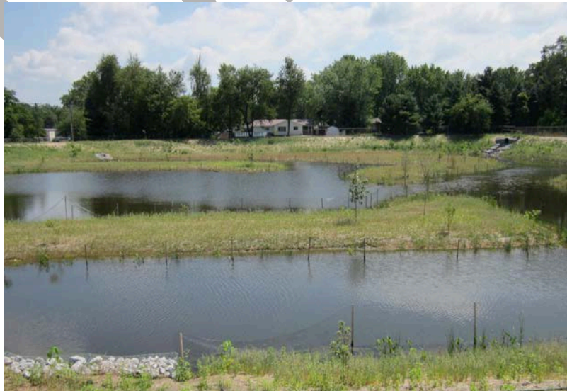
Figure X-4: Newly Installed Wall St. Bioretention Basin
