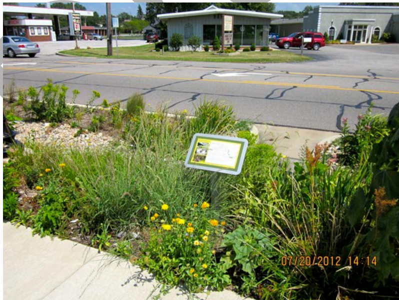
Figure X-2: Calumet Ave. Bioswale
