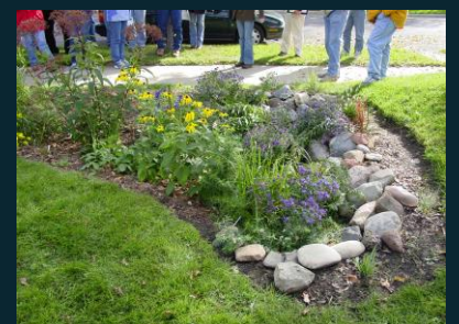
Rain gardens and bioswales are effective ways to manage and clean storm water on-site.
