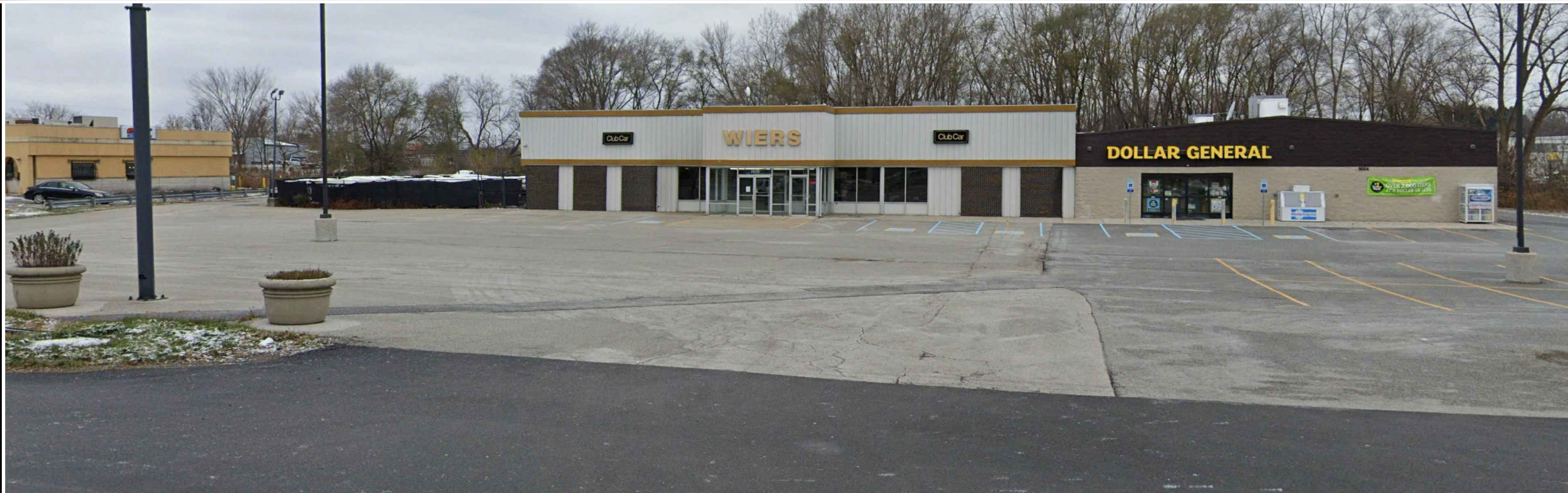
1 P-2 EXISTING VIEW FROM STATE ROUTE 2
